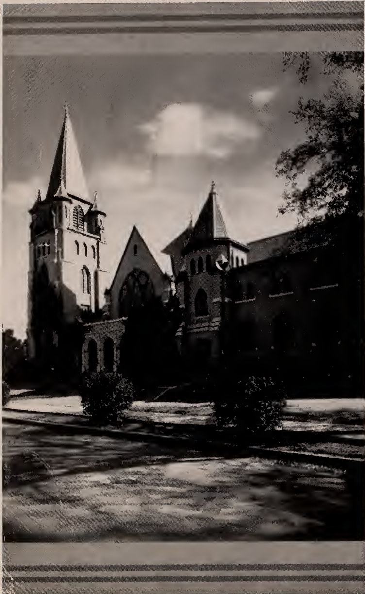
First Presbyterian Church, Gainesville, Texas
